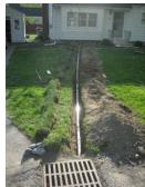
The water should be directed into your yard away from home sot that it does not puddle along the wall and seep back into your basement.
